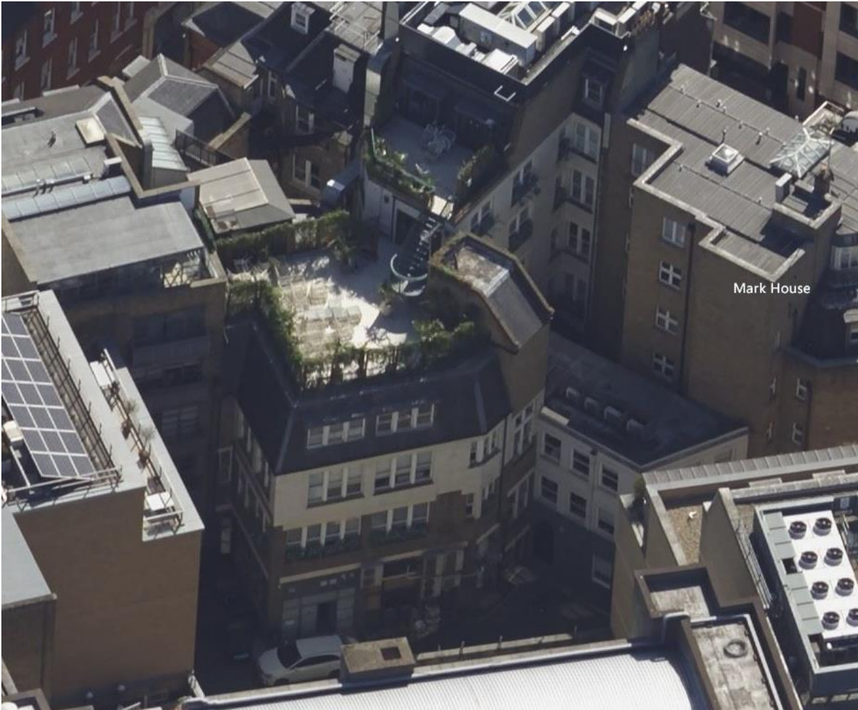
Aerial Photograph showing the terraces and the objectors windows –
